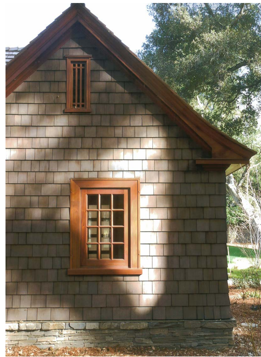
WALL AND ROOF SHINGLE EXAMPLE
