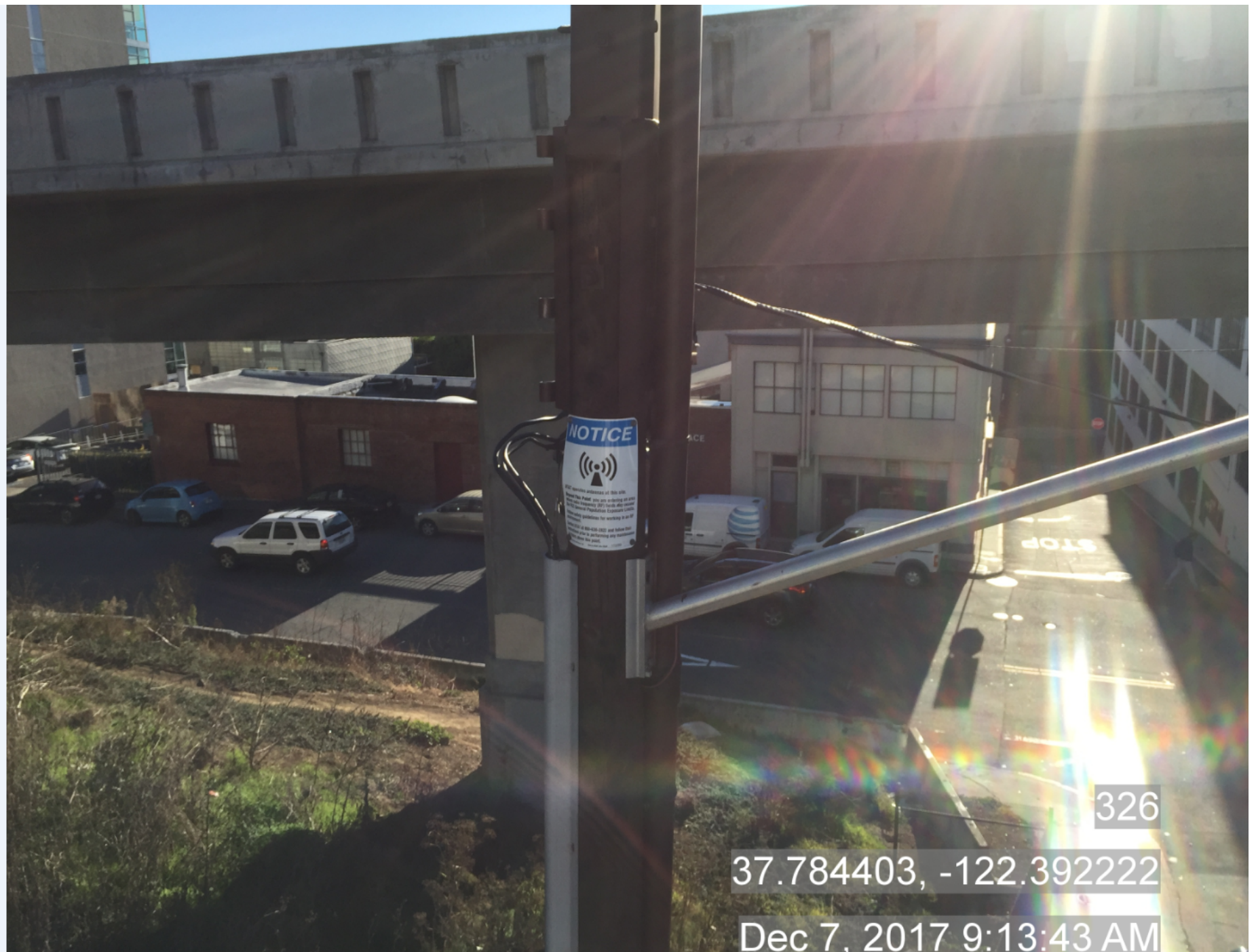
Example of proposed RF Notice Sign Located at or right below proposed antenna
