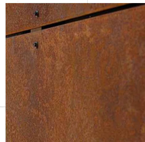
CORTEN STEEL PLATE AT ENTRY GATE AND GABION BENCH
