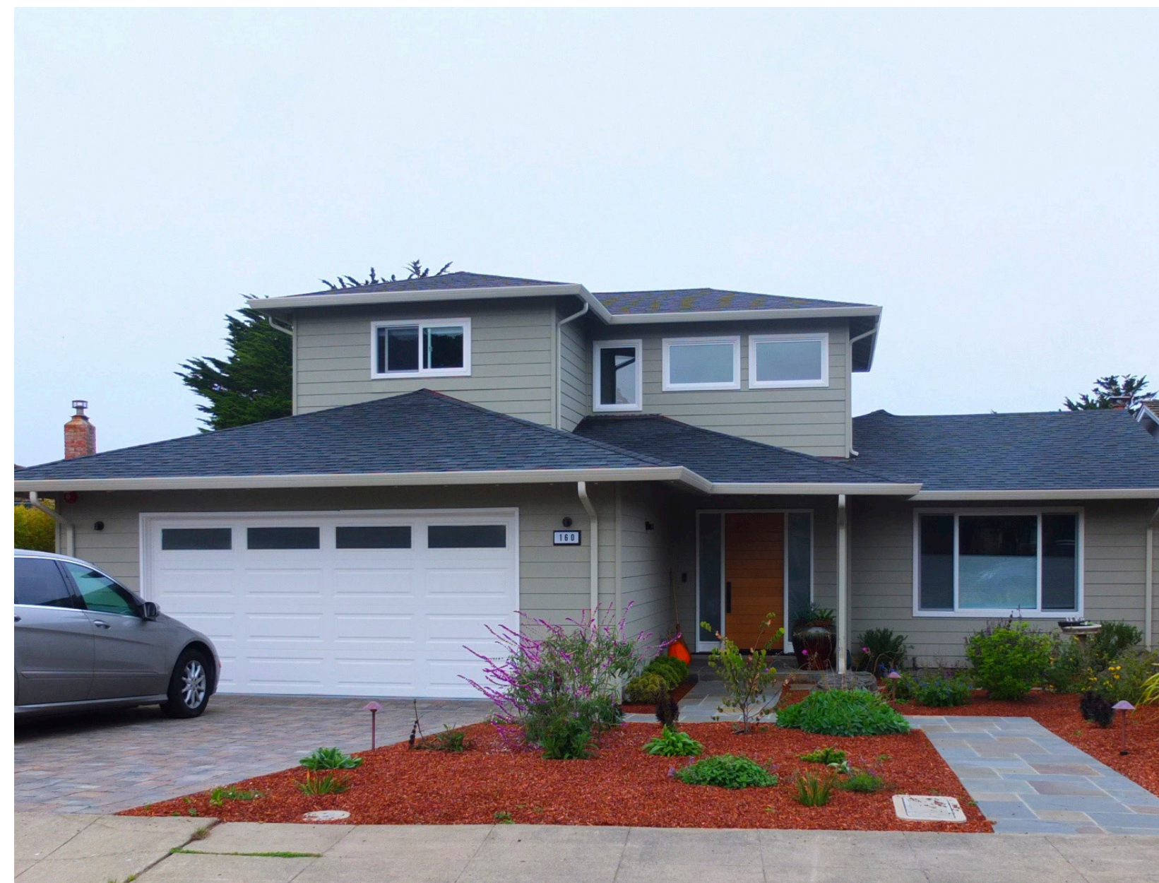
EXISTING ADJACENT HOUSE ON THE NORTH SIDE
