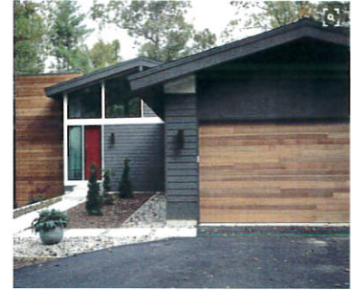
6. GARAGE DOORS: Natural wood Roll up doors - Western Red Cedar - Clr. polyurethane finish
