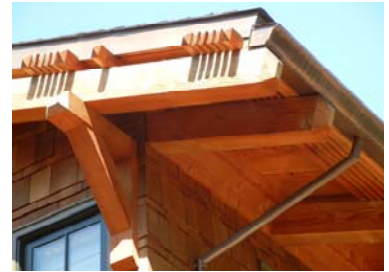
Building with copper flashing, gutter and drainpipe.
