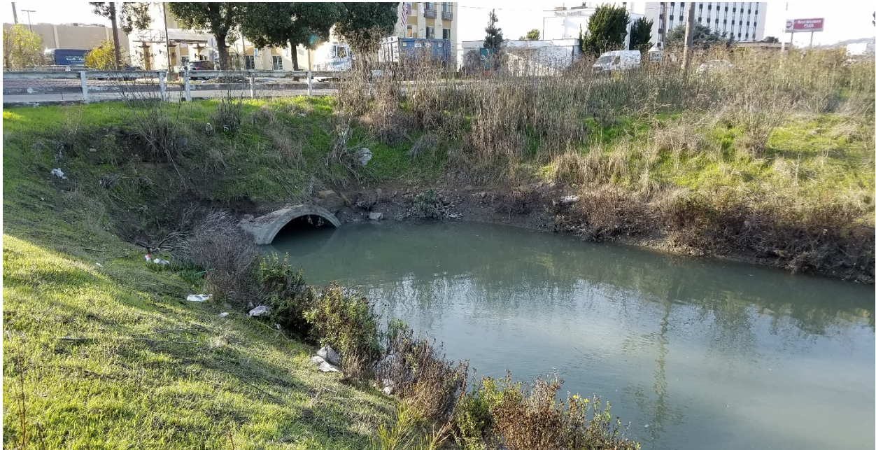
Figure 3-11. The culvert along Navigable Slough beneath South Airport Boulevard.
