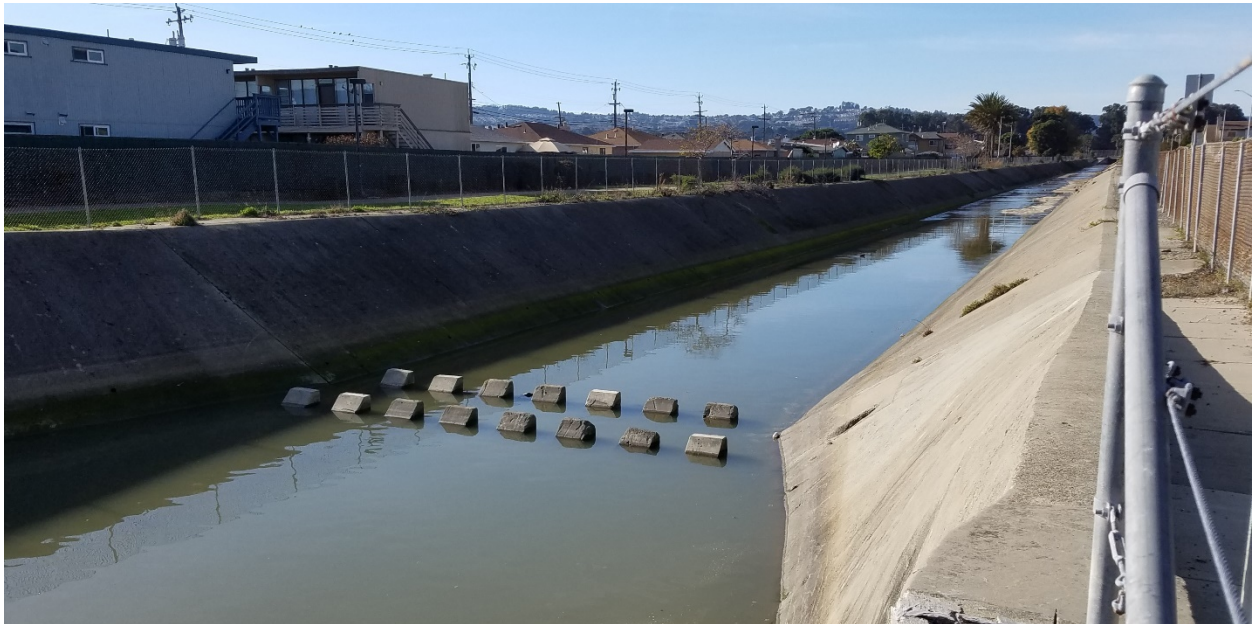
Figure 3-7. Energy dissipation structure located 300 feet above Spruce Avenue looking upstream.
