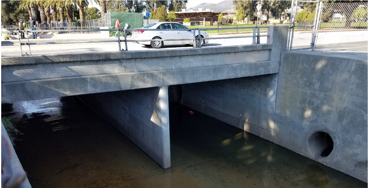
Figure 3-6. Orange Avenue Bridge, looking upstream, with the 36” storm drain shown (right).
