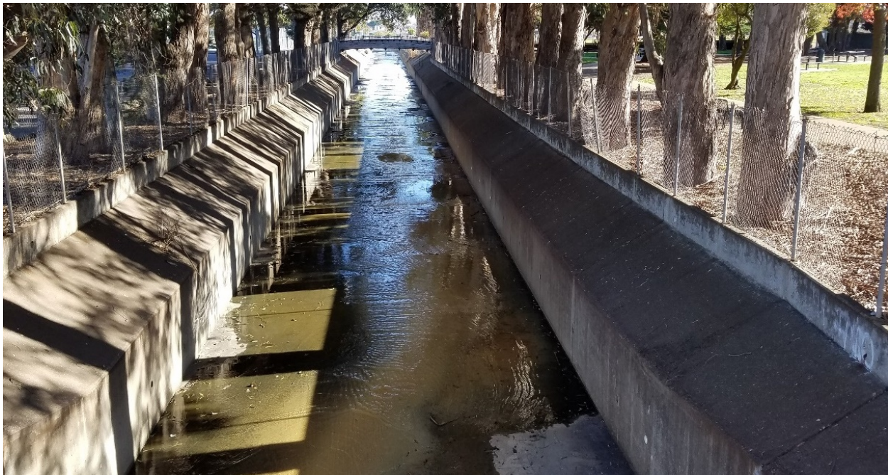
Figure 3-5. Compound trapezoidal-rectangular channel geometry in Colma Creek, looking downstream.
