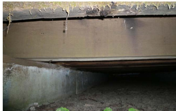
Figure 5 Joists and Grade Beam
