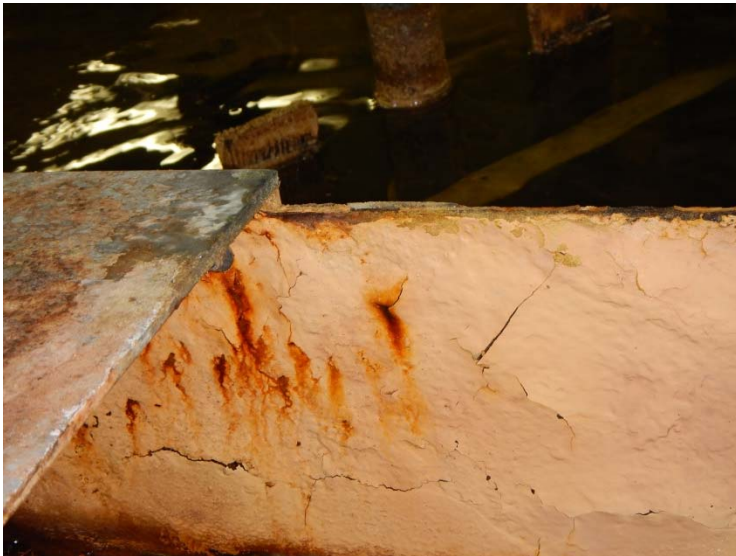
Figure 6: Flocculation Chamber Corrosion Resistant Paint
