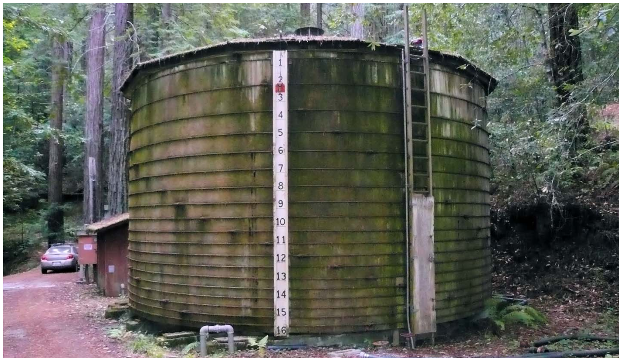
Figure 1 70,000 Gallon Redwood Water Storage Tank
