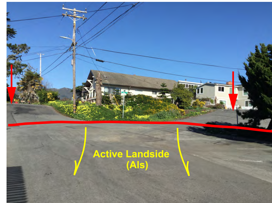
P1. North view from Distillery Restaurant across middle part of active landslide belt. Headscarp of AIs defined by rise in roadway between red line and arrows has retreated several feet toward southern perimeter of residence in distance over past 3 decades (note newer pavement repair where at left arrow that corresponds with the projection of southern part of the active landslide belt).
