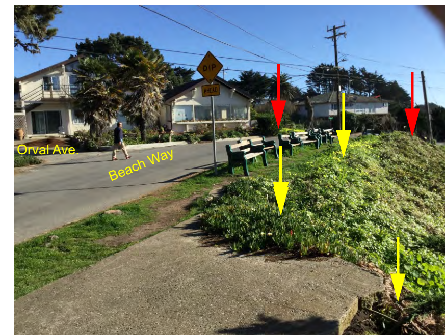
P2. Northwestern view along crown of headscarp in northern part of active landslide belt just north of the Distillery Restaurant (yellow arrows). Northward projection of active landslide scarp (red arrows) in P1 intersects the up to 40-foot high scarp of the stabilized landslide at the intersection of Orval Avenue and Beach Way. The presence of the remnant of concrete sidewalk from early 1900 subdivision speculation construction combined indicates scarp recession in this part of the active landslide belt has been relatively minor.
