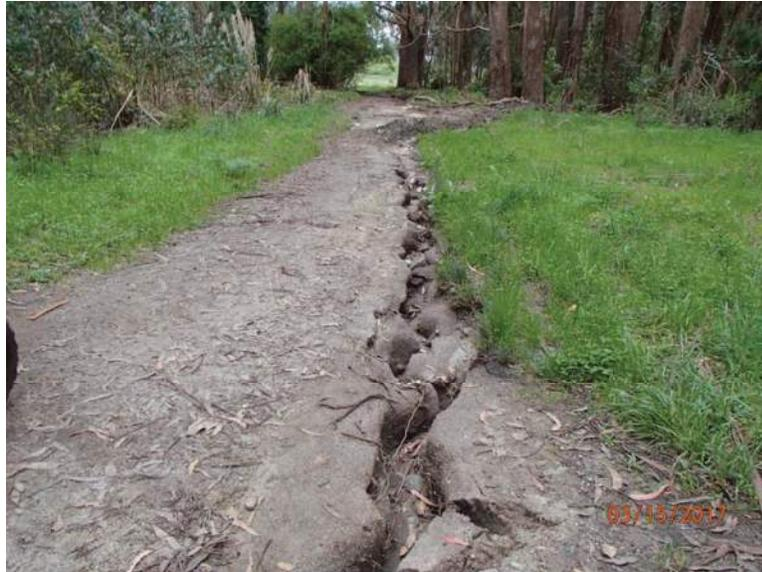
**Photo 3 (Meadow Trail):** View of active gully erosion along the Meadow trail. Combined diverted stream flow and concentrated road runoff are eroding the road surface along this native surfaced road.
