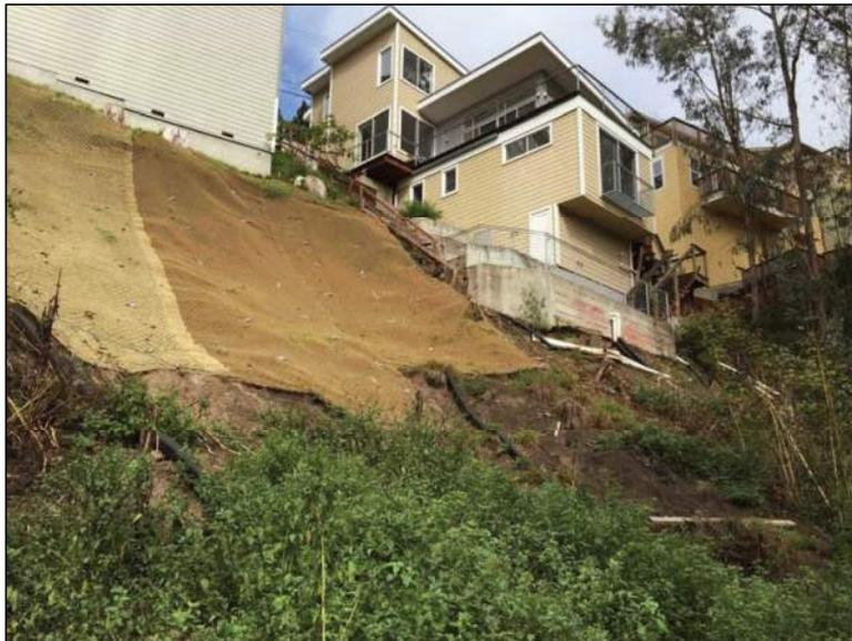
**Photo 20 (Site #41):** View of a hillslope failure and undermined residences upstream from Site #41. This area upslope extent of AOC 4 as discussed in the text of the report. This photo was taken from the outboard edge of the Fire Break Road upslope from the Upper Pond Legacy Road as shown on Map 2.
