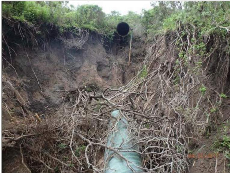
**Photo 17 (Site #40):** View looking upslope at the same disconnected downslope and active erosion as shown in the previous photo. The photo was taken from the base of the gully downslope of the headcut standing on top of one of the failed sections of culvert.
