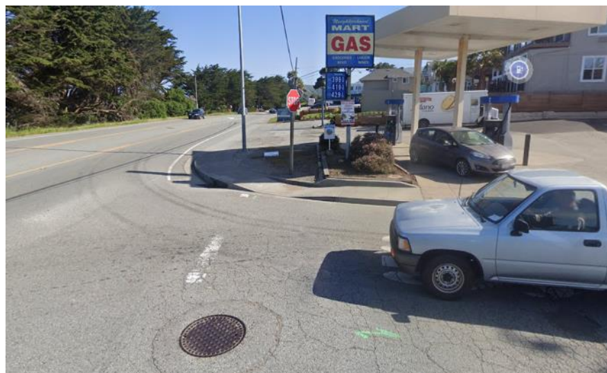
Example of a minor and stop-controlled intersection at Highway 1 and 8 th Street in Montara; 8 th street is the "minor and stop-controlled" street.
