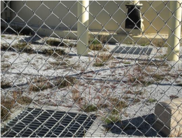
17. View of drains associated with the tanks
