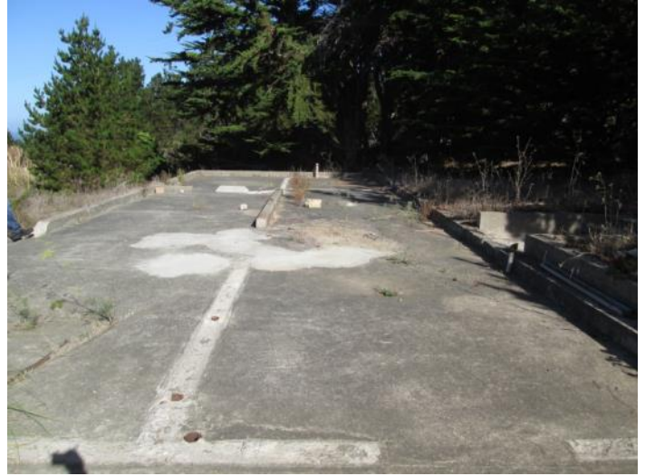
22. View of a concrete building foundation
