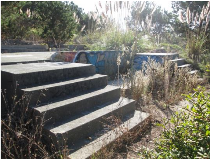
23. View of concrete stairs leading up to a concrete building foundation
