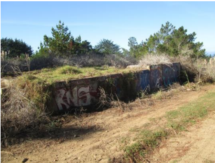
19. View of a concrete building foundation pad on the subject property
