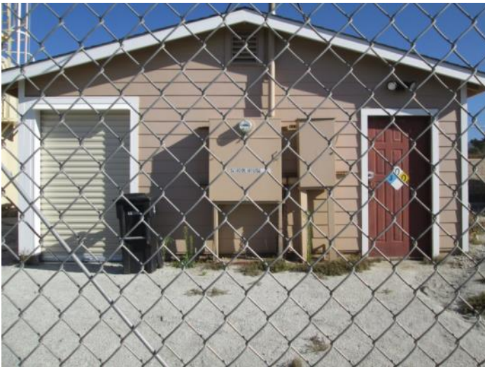
15. View of the building associated with the water tanks
